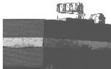
Fig 1.1 Building with a Cellular Antenna “crown”
