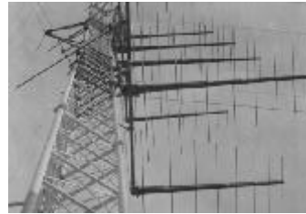
Fig. 5.12.2 Yagi antennas add substantial loading to the tower
