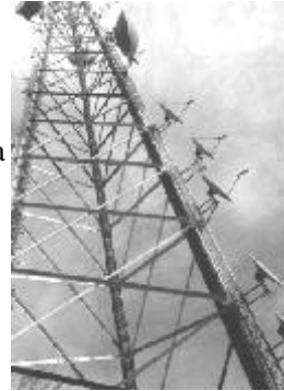
Fig. 5.12.1 Pager down-link dishes mounted low on a tower leg
